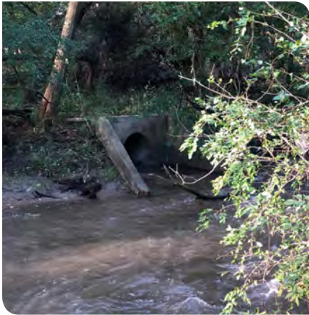
Chlorinated and saltwater can directly enter nearby streams if discharged into a storm sewer intake (ISWEP)
